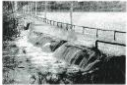
ROAD TO ISLAND PARK — The floodwaters of early November 1927 passed over the road in Island Park and washed most of it away.
