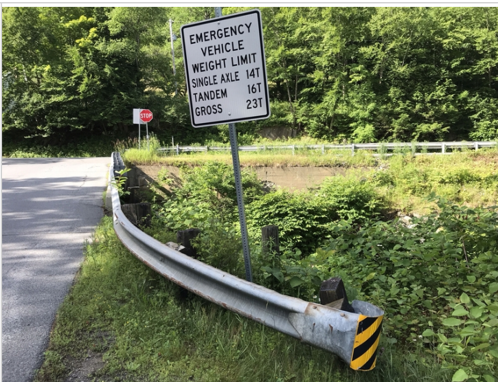
Approach rail to abutment 2 wingwall 3
