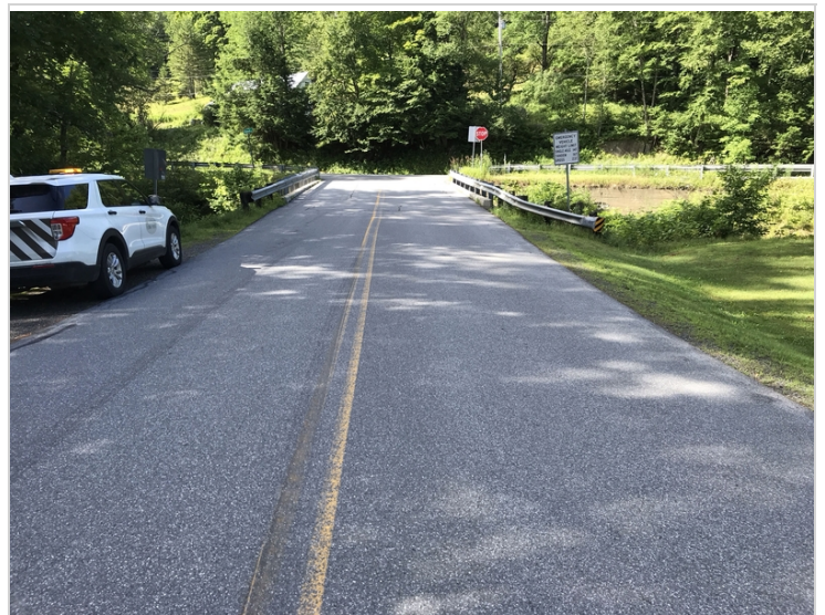
Abutment 2 approach (East)
