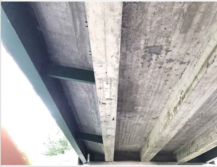
Soffit & superstructure bays 3 & 4 facing abutment 1
