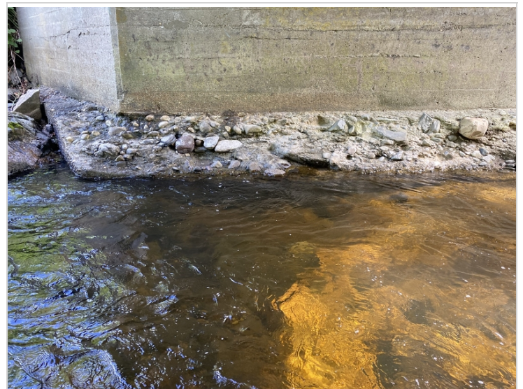
Footing along Abutment #2
