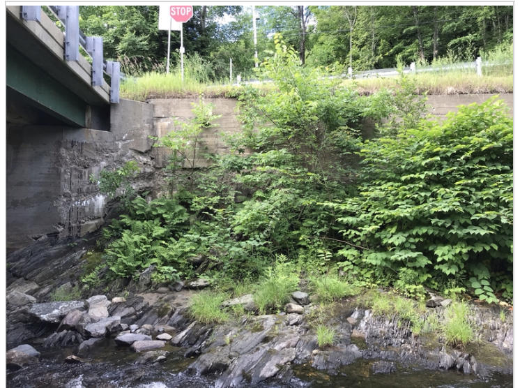
Wingwall 1 & upstream retaining wall
