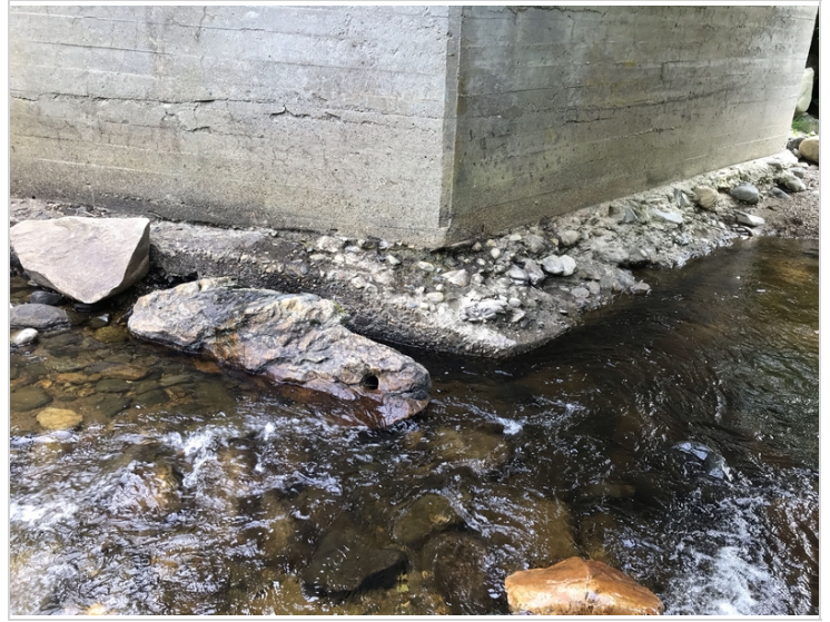
Wingwall 3 & abutment 2 footing
