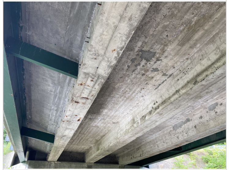
Concrete T-Beams from Abutment #2
