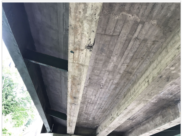
Soffit & superstructure bays 1 & 2 facing abutment 2
