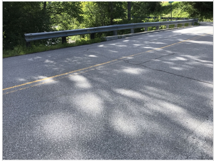
Downstream approach & bridge rail
