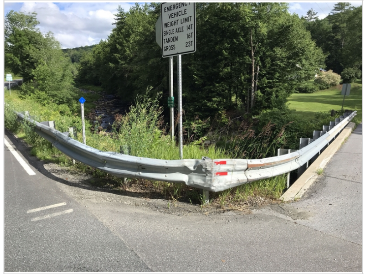
upstream approach & bridge rail at abutment 1 wingwall 1
