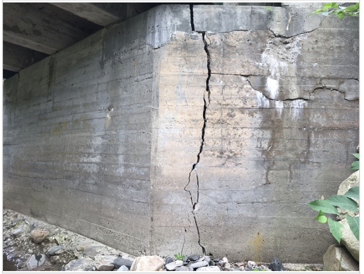
Wingwall 4 at abutment 2
