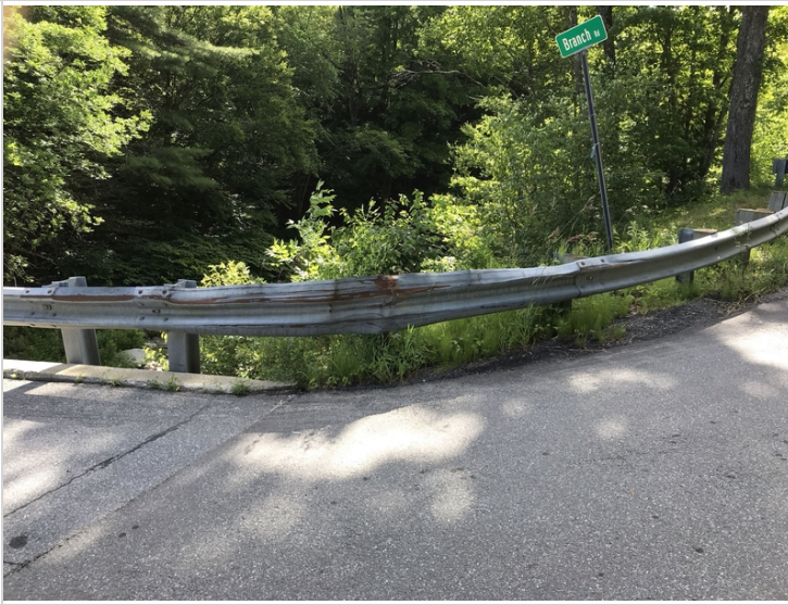
Downstream approach & bridge rail at abutment 1 wingwall 2
