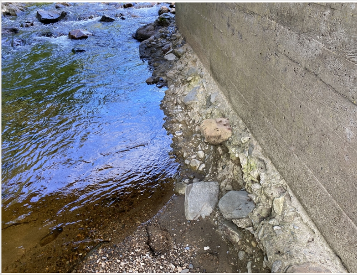
Footing along Abutment #2
